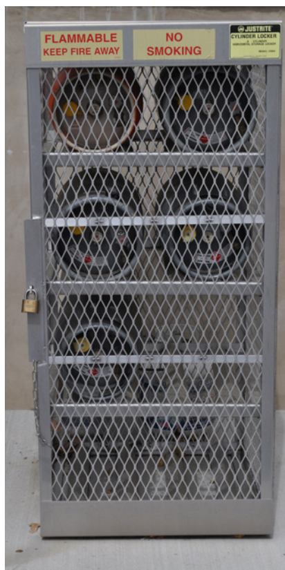
Figure 3.13. Approved propane cage.
