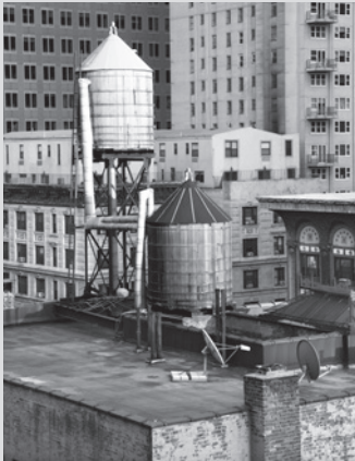
Figure 2.12. Workers must be protected from fall hazards at roof edges. Parapets must meet minimum height requirements to be considered adequate fall protection.
