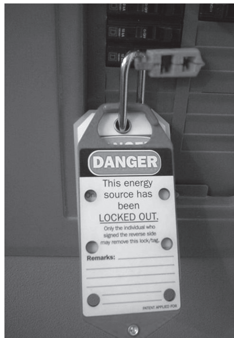
Figure 2.19. Never bypass a lockout/tagout device that someone else has placed on a piece of equipment.
