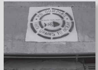
Figure 2.18. Know the restrictions before putting anything into a storm drain.
