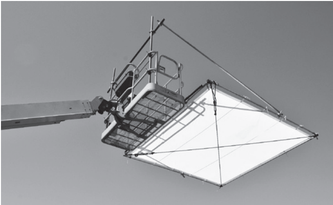
Figure 4.5. Equipment can be blown away during high winds.
