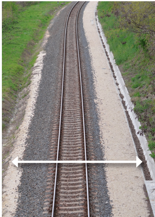
Figure 2.21 A railroad right-of-way is property owned by a rail company that runs the length of their tracks. The width of the right-of-way (shown by the arrow) can range from 25 feet to over 100 feet.
