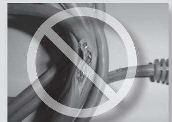
Figure 6.2. Damaged insulation can expose people to injury from burns and electrical shock, and can lead to a short circuit, overheated wires, sparks, and fire.
