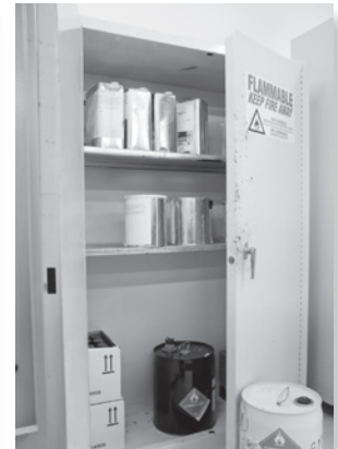
Figure 6.5. Be sure flammables are stored in an appropriate cabinet.
