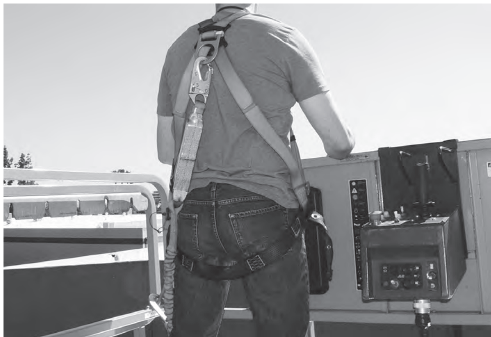
Figure 4.2. Personal fall protection, such as a body harness, is required to be worn by occupants of aerial platforms, and is recommended for occupants of scissor lifts.
