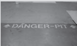
Figure 4.12. Pits and tanks may be marked on the floor and identified on posted floor plans.
