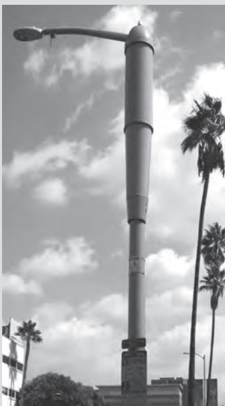
Figure 5.3. Smart poles combine street lighting with other technology. Observe the clearance distance marked on the pole.
